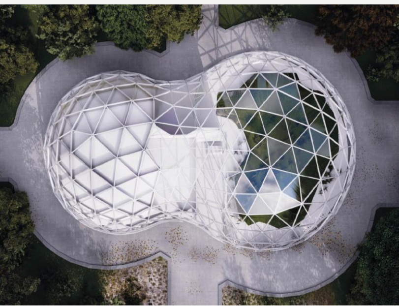
The same roof from above: two intersecting shells over one plan.
