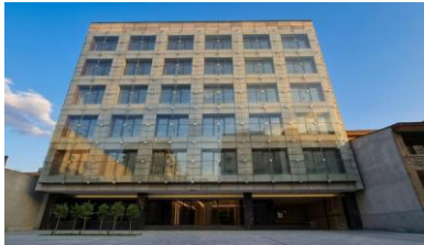
06 B CABLE-SUPPORTED CURTAIN WALL
