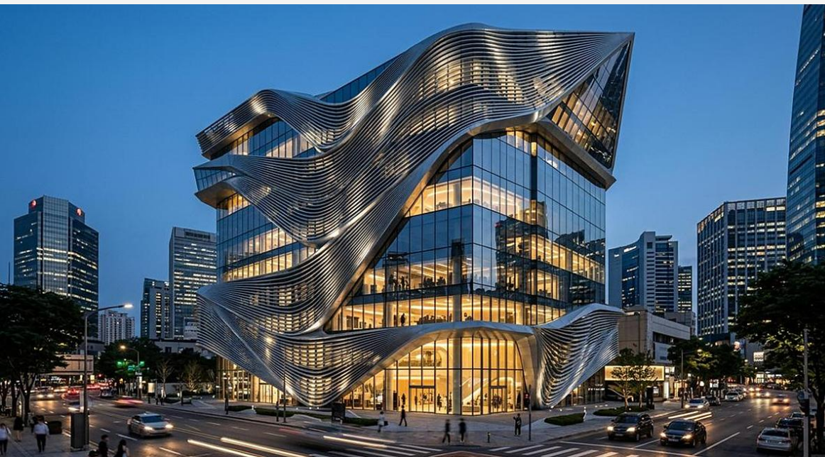
Extruded aluminium blades set as the elevation itself.
