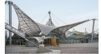
05 B CABLE STRUCTURES
