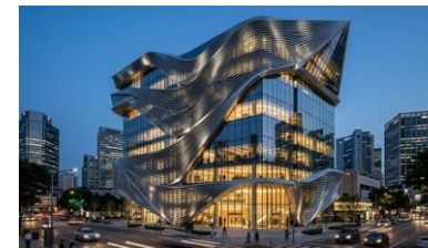
14 C ALUMINIUM LOUVRE FAÇADE
