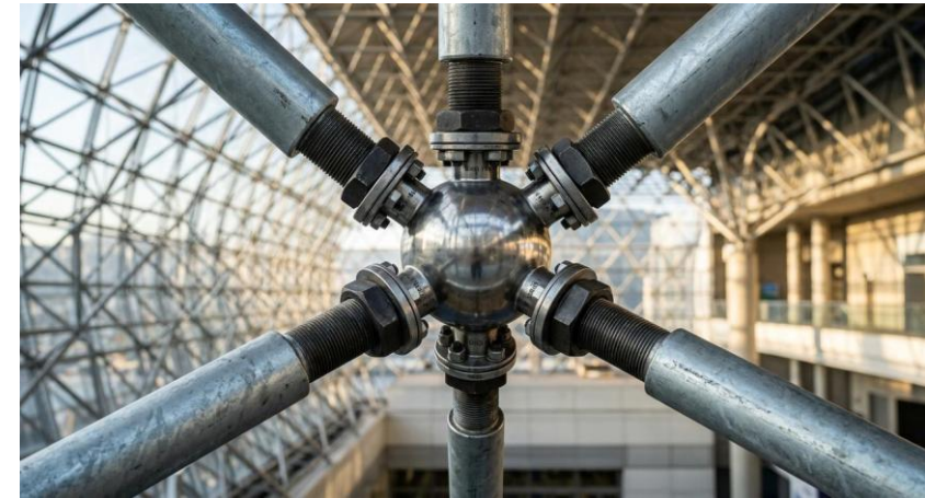
Erection in progress, and a typical node. Members and connectors arrive finished; assembly is repetition rather than fabrication.
