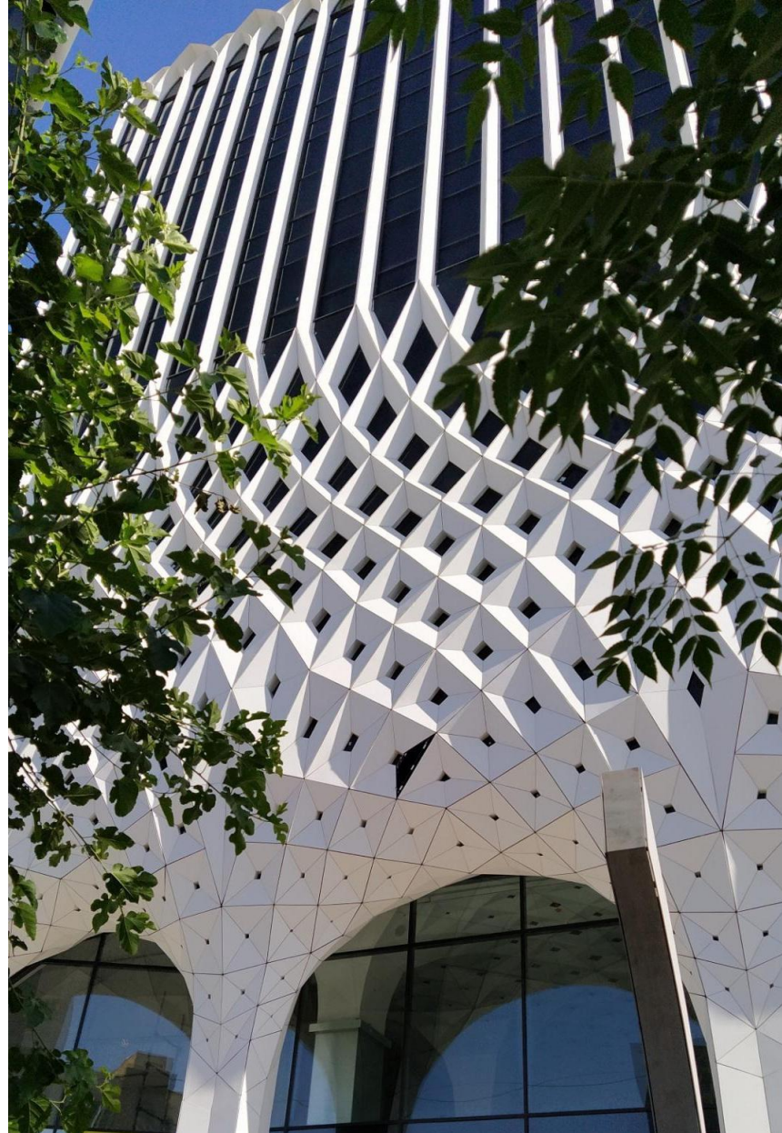
Parametric shading structure — geometry rationalized into a repeatable node set.
