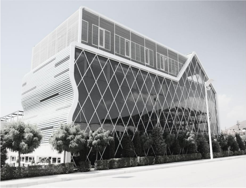
The completed louvre field at Pardis Technology Park.
