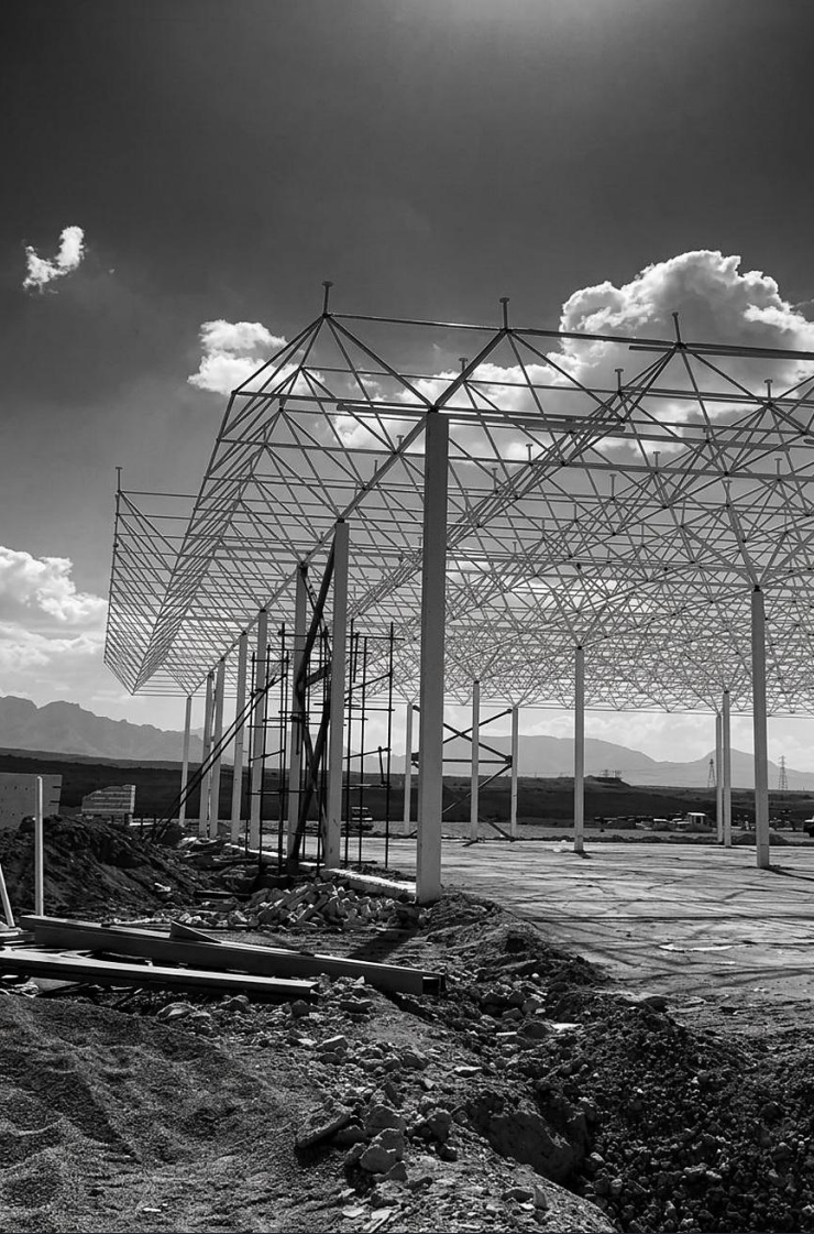
Arian Motor Factory — space frame erection, Arak.
